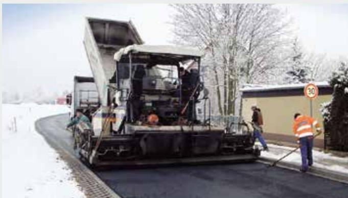
Likewise, risks to be fined for failed compaction rise. **aspha-min®** significantly improves the workability and compactibility of the asphalt mix. This leads to improved compaction results for thin layers, demanding mixes and under adverse weather conditions. Since workability is guaranteed at temperatures as low as 100 °C, the time frame for paving under such circumstances is clearly extended.
